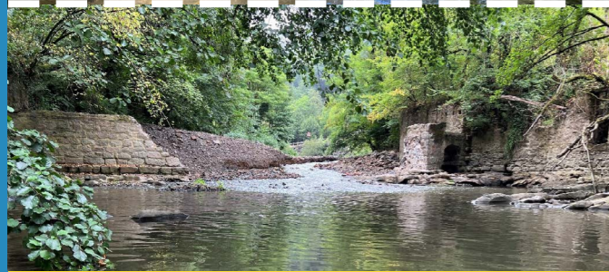
SAN PRUDENTZIO DAM – DEBA RIVER – SPAIN © Gipuzkoa Provincial Council
